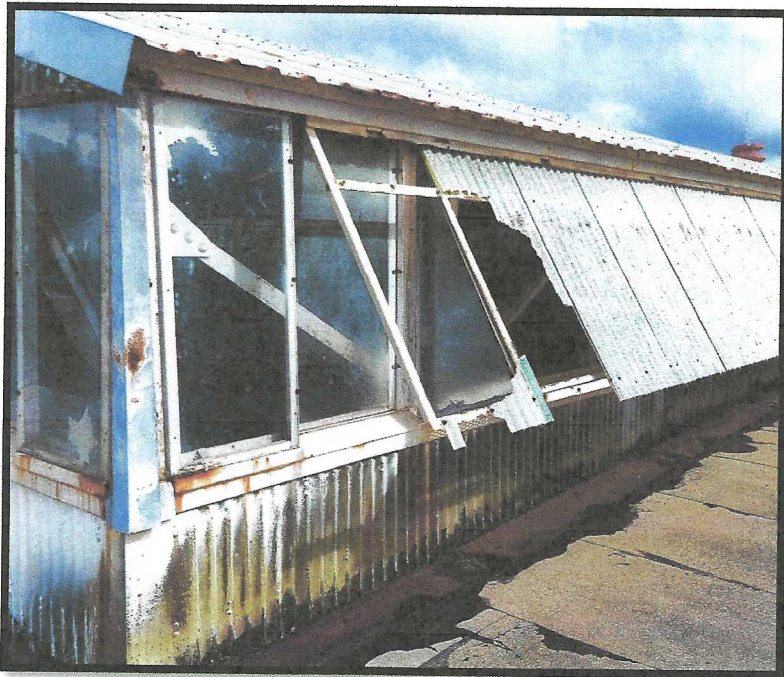
Translucent panels on the monitors were designed to provide additional light to enter the Hangar and protection from the rain. Many of the panels have been damaged and will need to be replaced with a modern transparent polycarbonate plastic.
