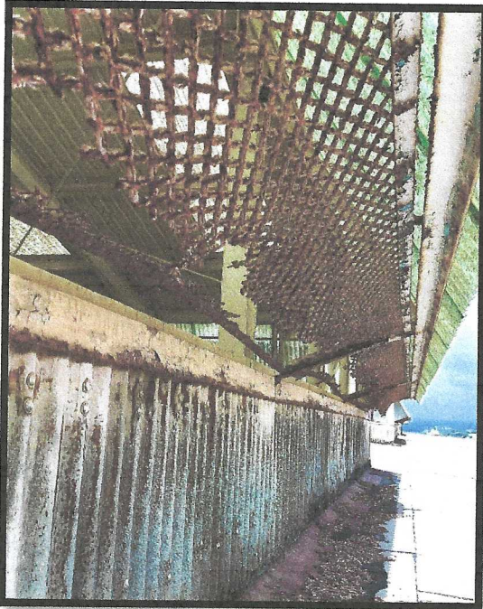
Wire mesh around the monitors, which allow hot air to escape and cool air to enter, are completely rusted and need to be replaced.
